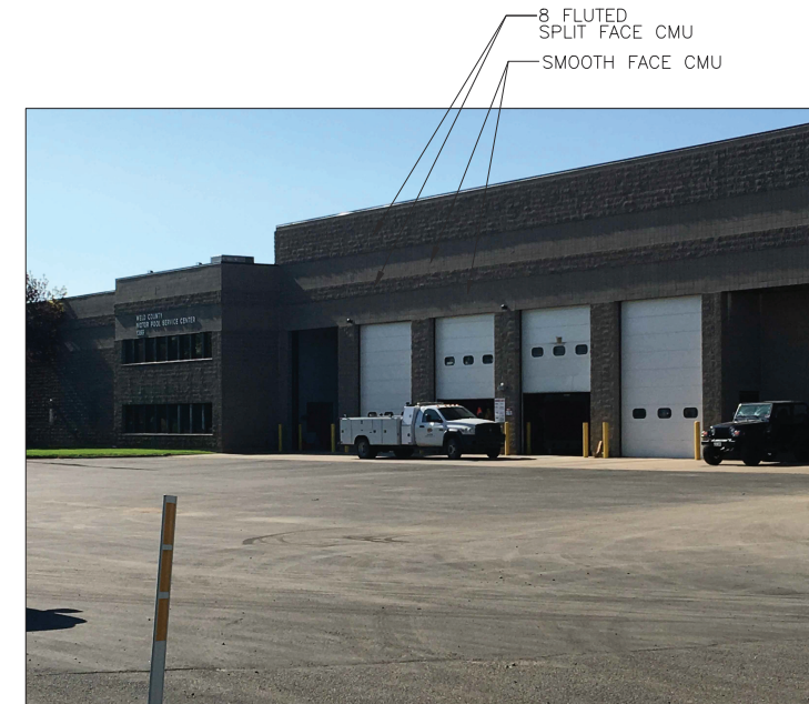
WELD COUNTY MOTOR SERVICE CENTER
