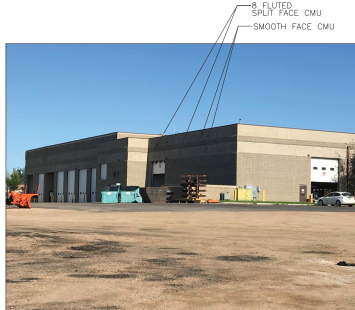
WELD COUNTY MOTOR SERVICE CENTER
